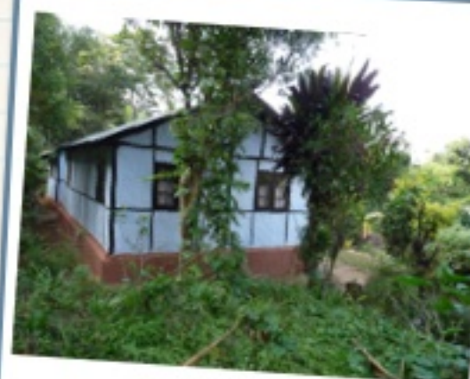
Village house built with woven bamboo, mud and timber beams
